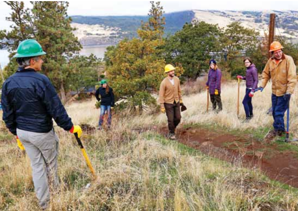
Steve Kruger, executive director of Trailkeepers of Oregon, in yellow helmet, working with trail volunteers.
