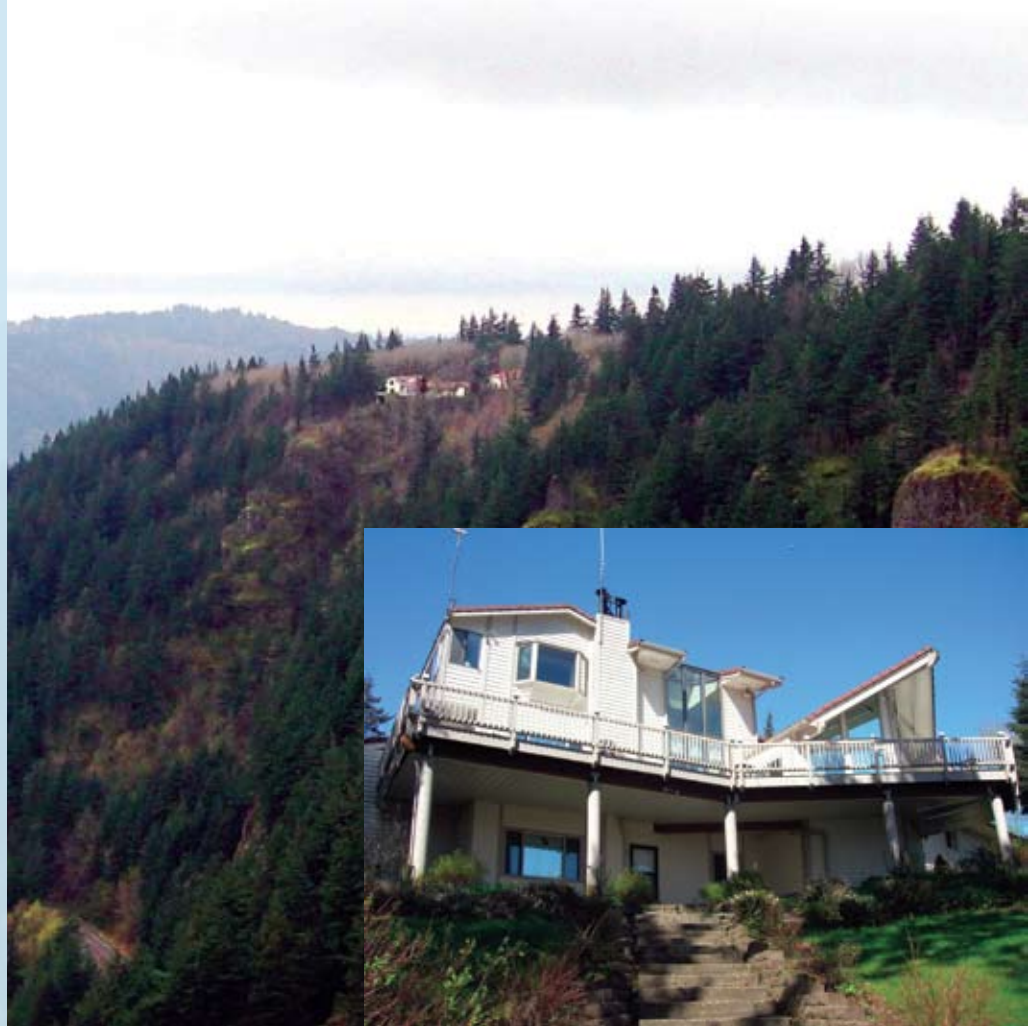
The trophy home and barn on the Cleveland property at Cape Horn will be deconstructed this summer. Photo: Dan Huntington
