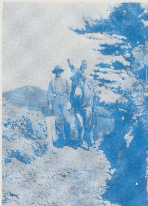
"Trail Burro and Assistant." Construction of the Beacon Rock Trail, circa 1917 from Rodney Glisan Album, Mazamas Library, Oregon Historical Society.
