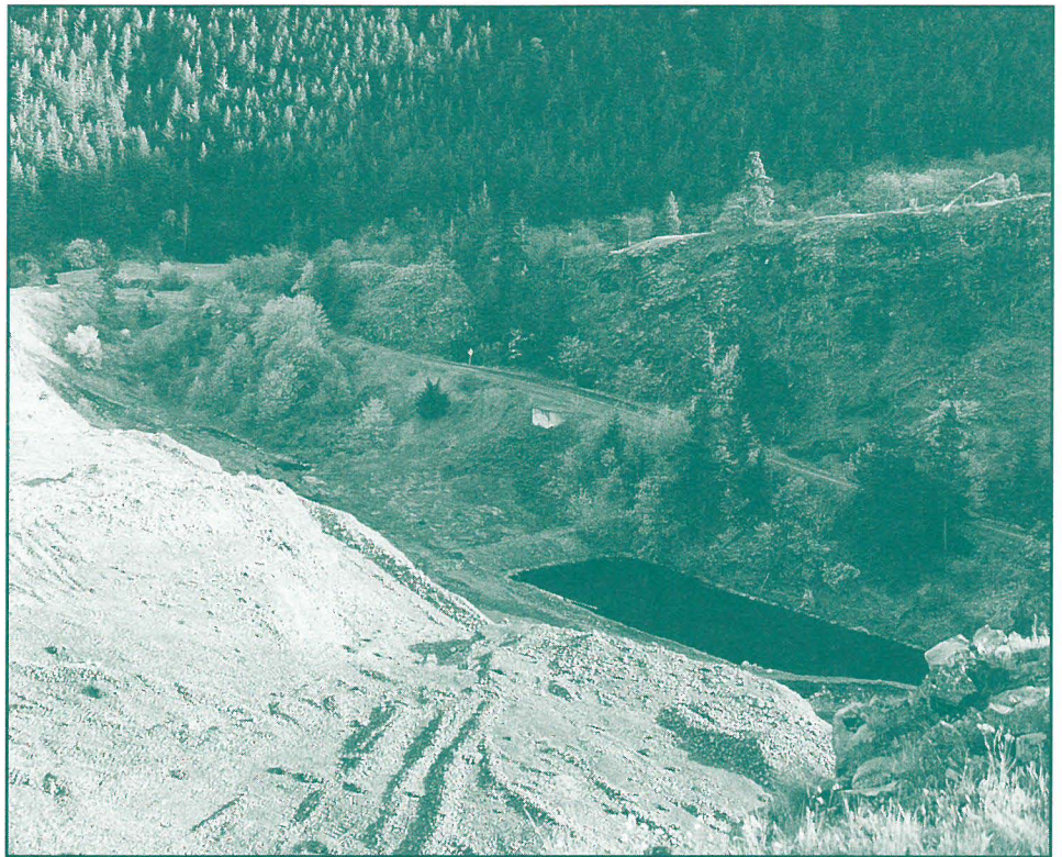
The ravaged ground of the East Pit Quarry is a stark contrast to the forests and fields along the Historic Columbia River Highway. Hood River County wants to keep the quarry open despite a decision that the quarry, clearly visible from the Historic Highway, is inconsistent with the National Scenic Act.
